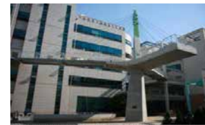
The world's first UHPC pedestrian cable-stayed bridge Image by Byung-Suk Kim
