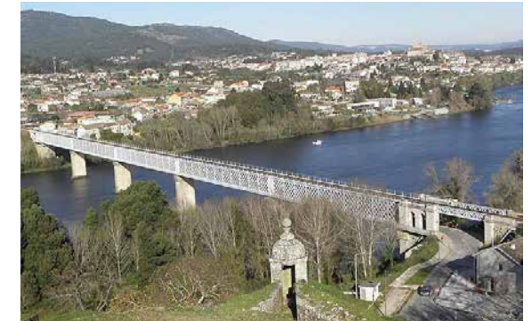
Valença Road-Rail Bridge - 1885
