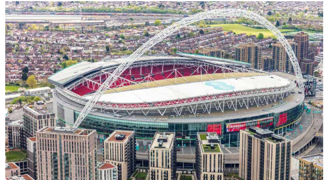
Wembley Stadium (UK)
