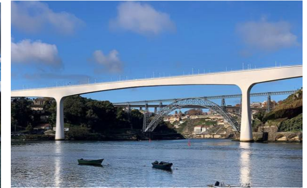
São João Bridge - 1991
